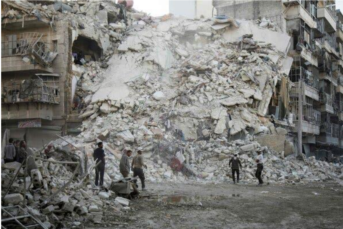
A building destroyed by air strikes in Aleppo, Syria, in October 2016. Credit...Karam Al-Masri/Agence France-Presse — Getty Images
